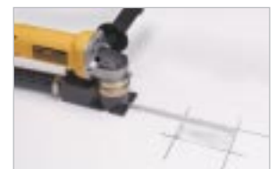
Cut the Wiring Chase
